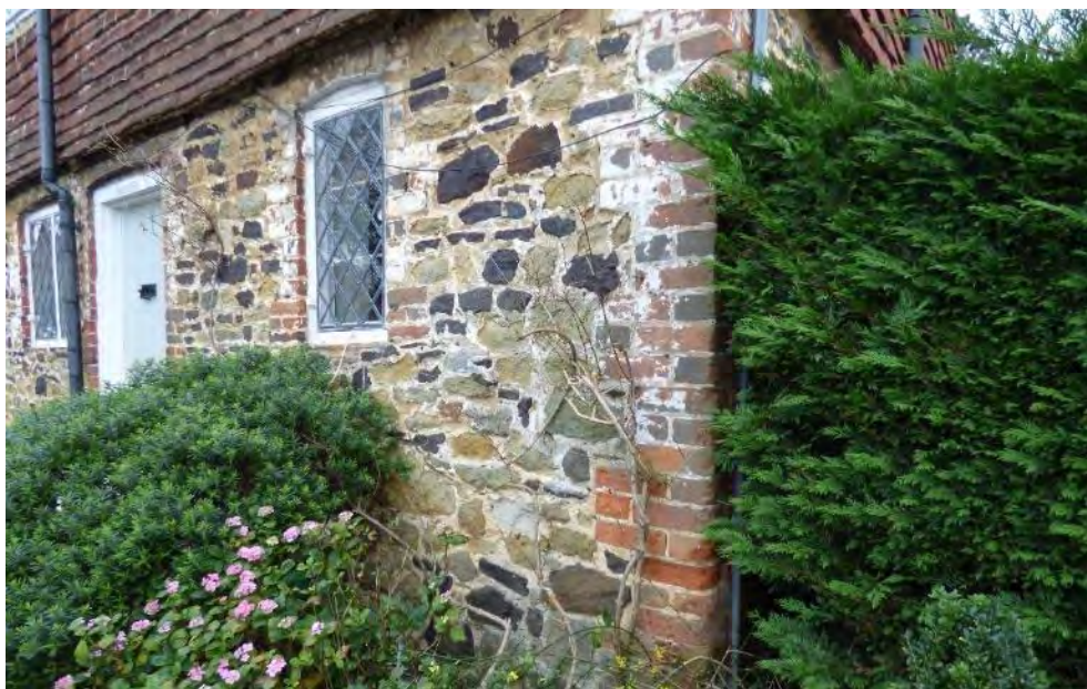
Figure 20: Wall with Greensand stone and ironstone typical of Limpsfield Village.
