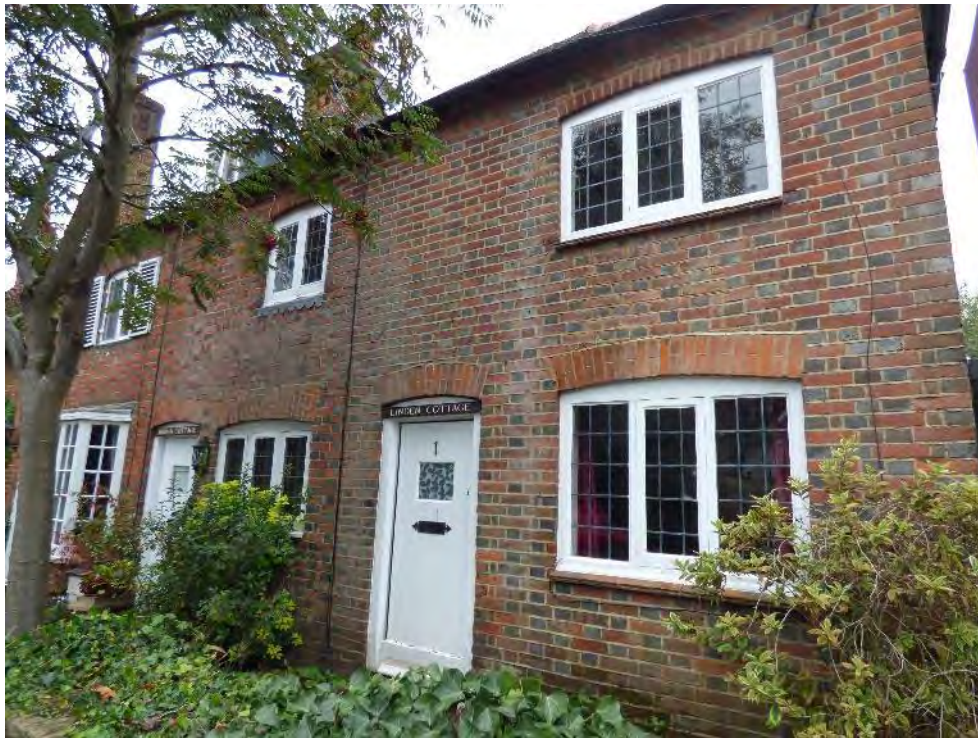
Figure 41: An example of blue header brickwork within the Conservation Area.
