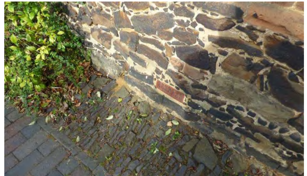
Figure 40: Ironstone paving and galletting on a property on the High Street.
