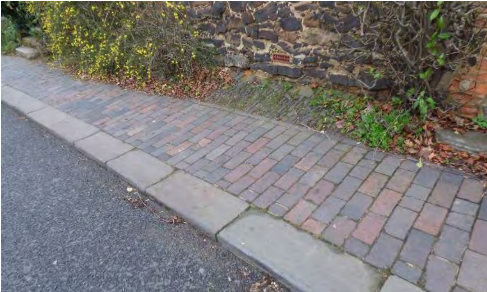
Figure 45: Historic wide sections of sandstone paving with brick paviours.
