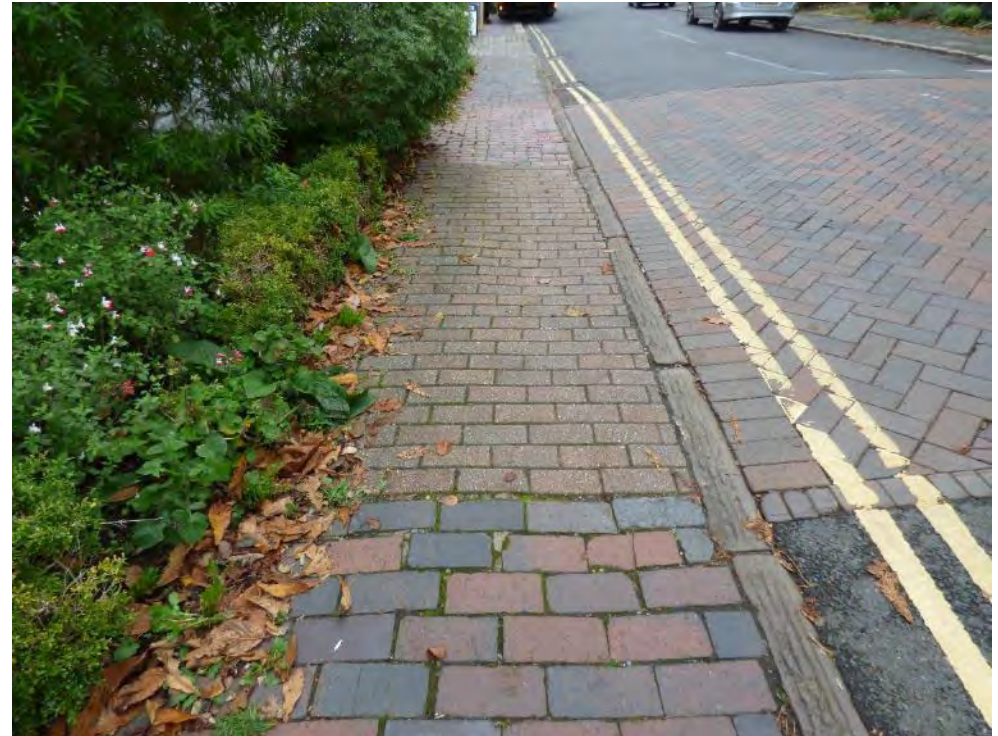
Figure 46: Replacement sandstone kerbstones with a mix of original and replacement brick paviours.
